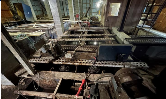
Wastewater Treatment Plant Building Determined unsafe for entry and non-functioning
